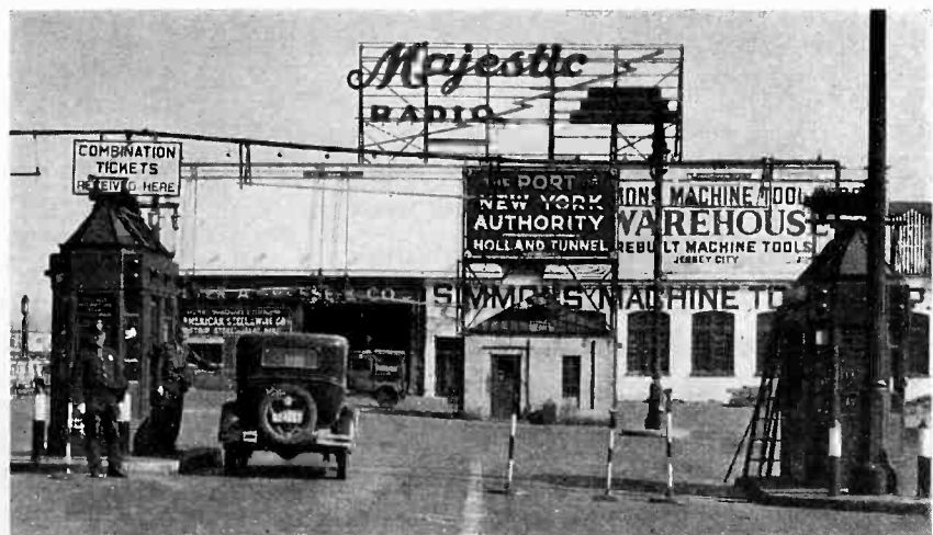
Trucks more than 12 ft. high approaching this Holland Tunnel entrance, intercept the 33-ft. beam controlling a photo-cell which rings a warning bell in the ticket-booth
